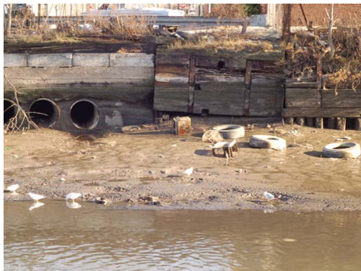
Combined Sewer Overflow along the banks of the Gowanus Canal. Photo Credit: Eymund Deigel
