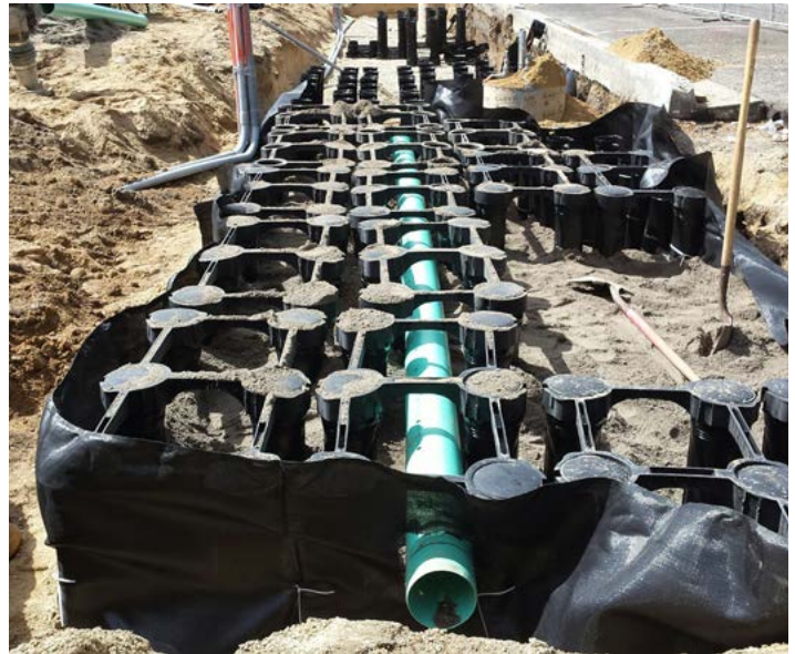
Silva Cell installation. Source: Deeprout
