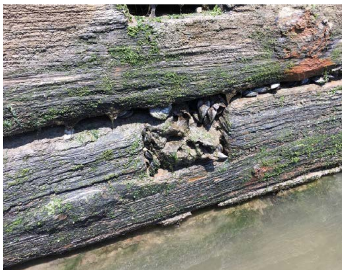
Geukensia demissa, or Atlantic Ribbed Mussel populates a bulkhead constructed of wood cribbing, 2018
