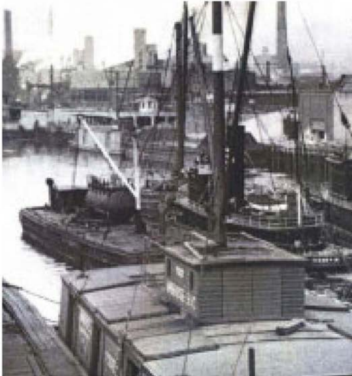
REGISTER THE VERTICAL STRUCTURES
