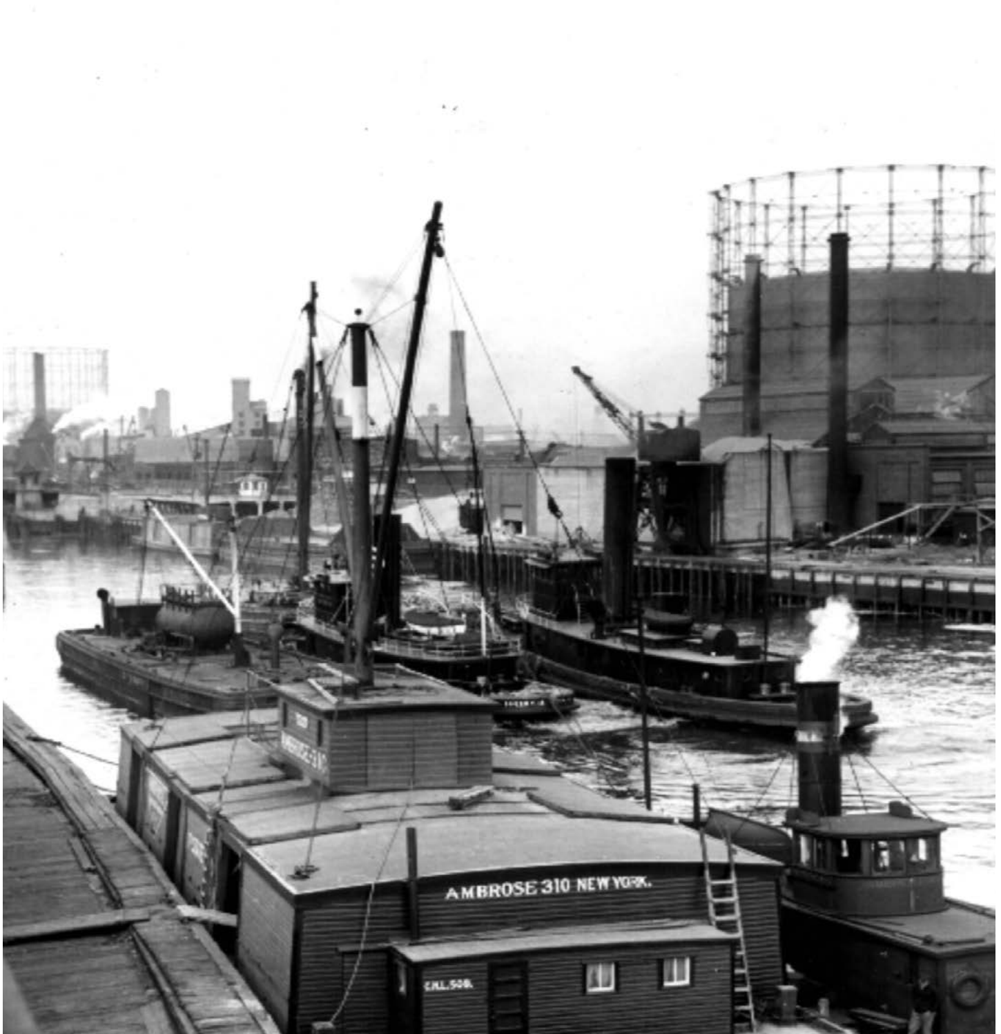
Metropolitan Gas Works from Canal facing North, 1930's, National Grid Archives
