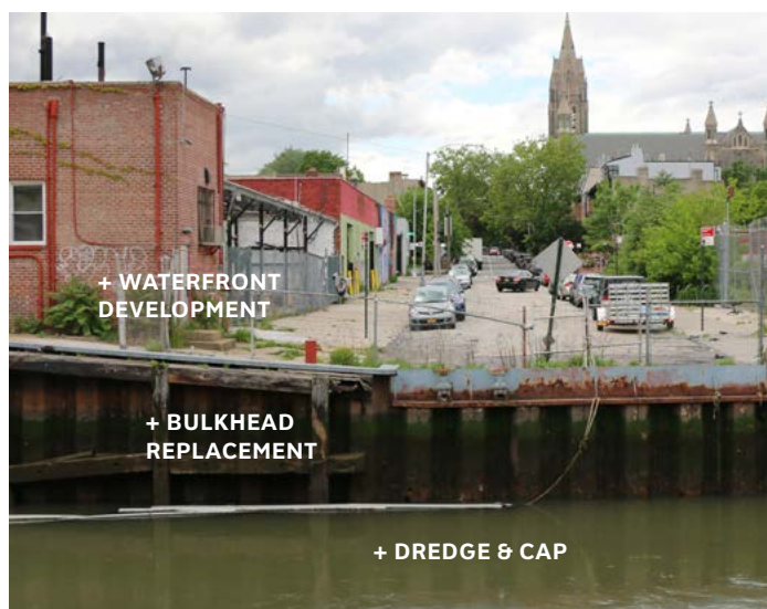
The Superfund clean-up will dramatically alter the shoreline by replacing most bulkheads with vertical steel sheet pile.
