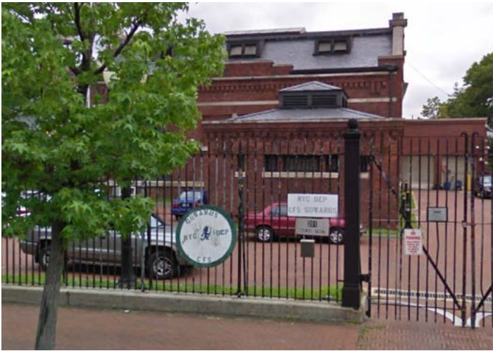
Pump House existing condition: there is currently no public access to the pump house or the Head of Canal.
