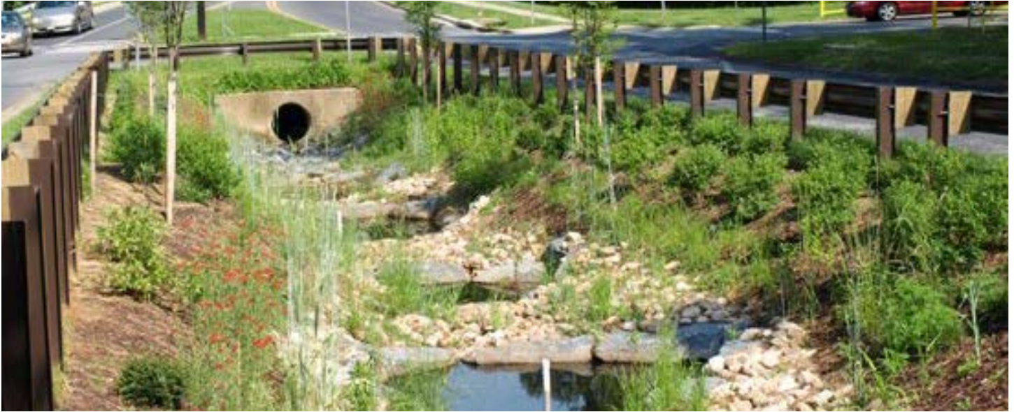
Stepped wet swale. Source: Virginia Association of Soil and Water Conservation Districts
