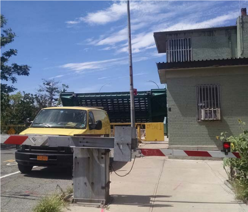
The Union Street Bridge undergoing maintenance to ensure operations for regular opening during the Superfund clean-up
